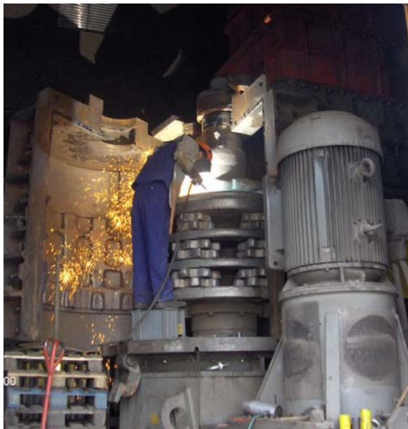
Figure 2: Hammer mill during maintenance activities.
